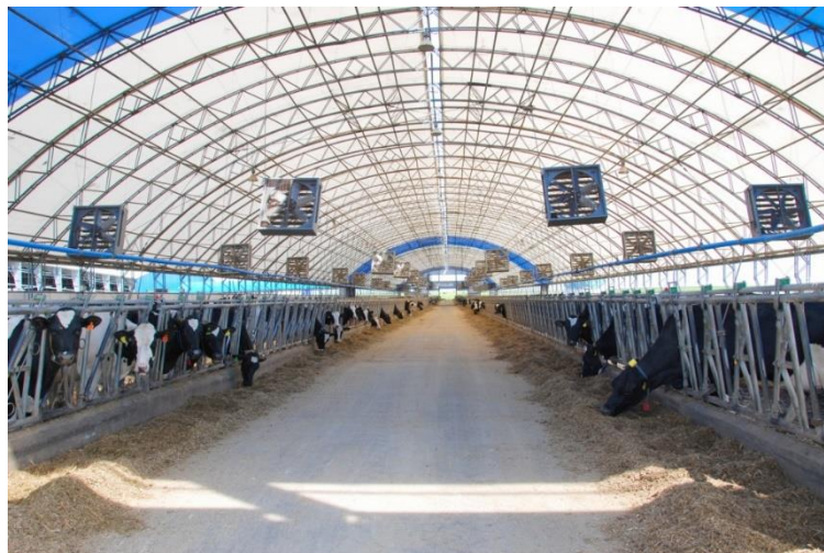
Fig. 1. Uninsulated cowshed of the hangar type with an awning coating
