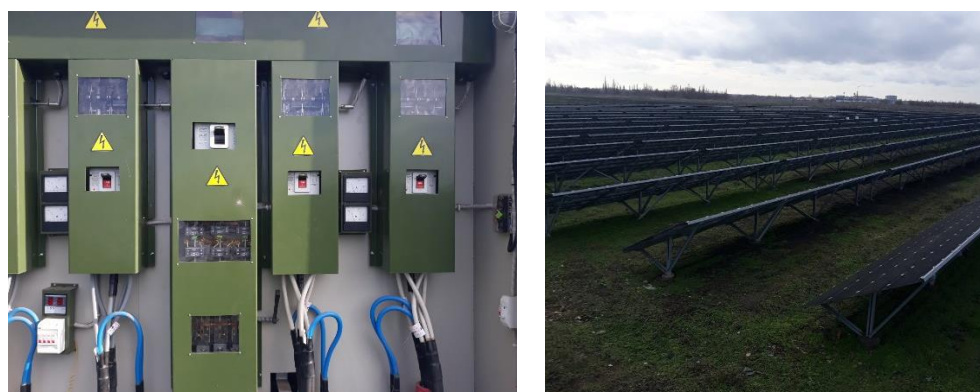
Figure 4. The solar PV power field (Mykolaiv province).
